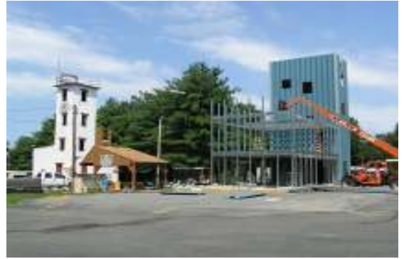
The new Fire Training Building nearing completion
